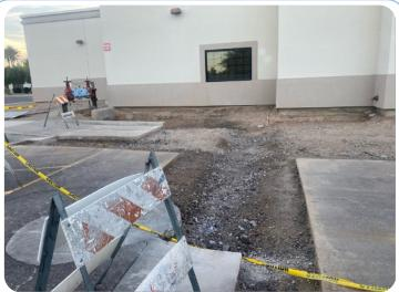
This is repair work on the drainage along the fire lane near the FLC. When it rained, a "lake" would form rather than drain away. Along with this repair, the entire parking lot was crack sealed and slurry coated. This is part of our part of our on-going campus repairs and maintenance. Thank you for your faithful giving of your tithes and offerings so we can maintain our facilities and beautify our campus!
